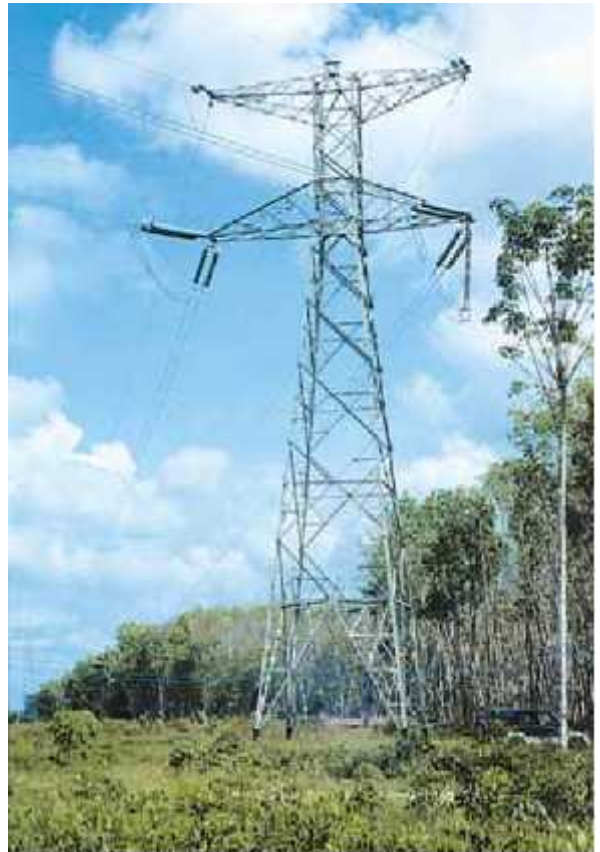
Fig. 5.6.1-1: DC transmission line (bipolar tower 300 kV link)
